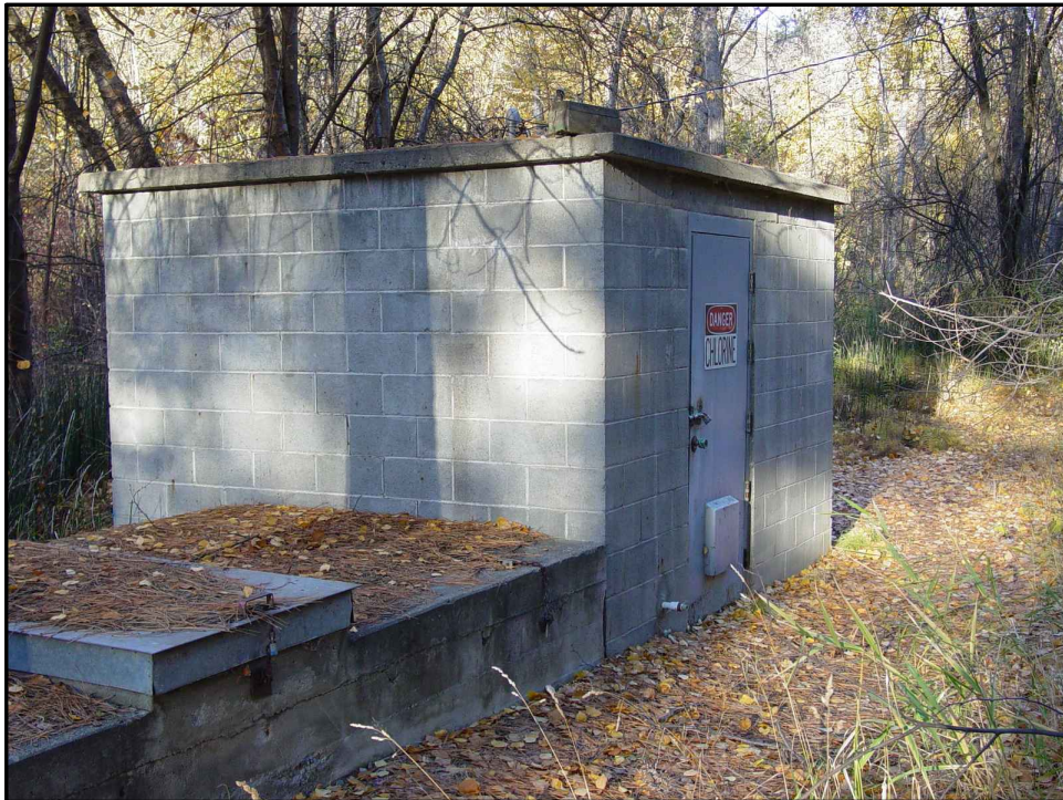
WATERCRESS SPRINGS CHLORINATION BUILDING
